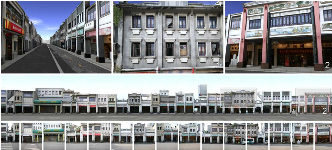
Figure 1: A few façade modeling examples from the two sides of a street with 614 captured images: some input images in the bottom row, the recovered model rendered in the middle row, and three zoomed sections of the recovered model rendered in the top row.
